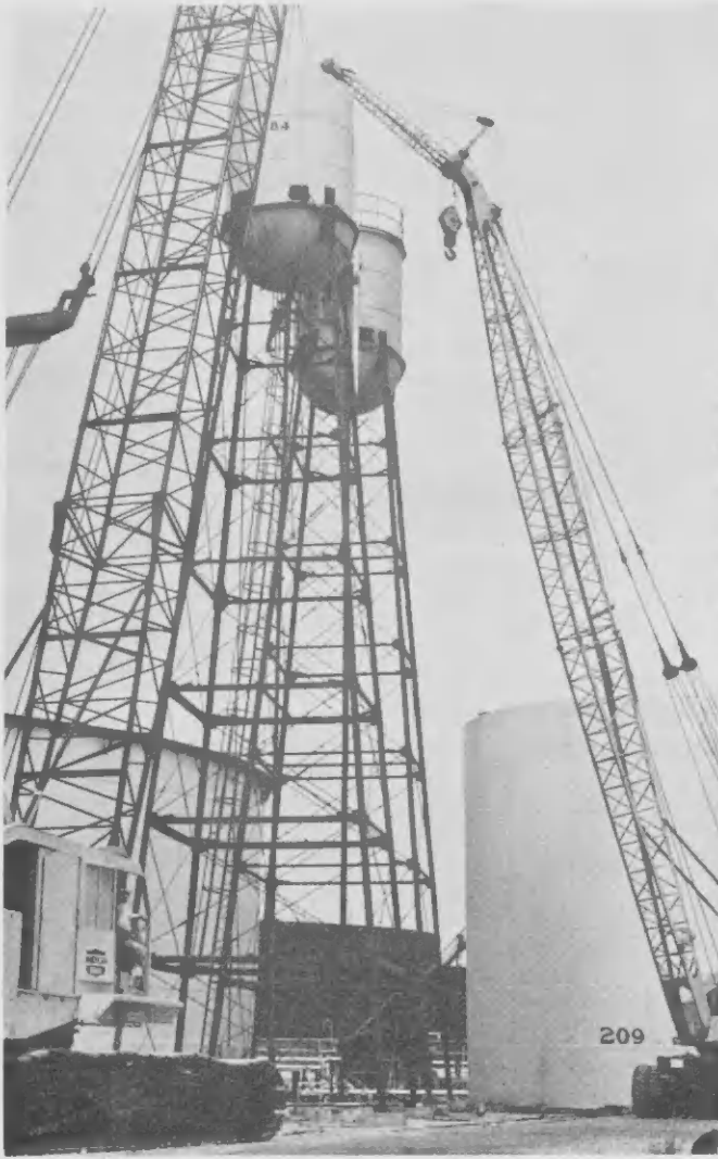
THREE WATER tanks were removed from the refinery skyline recently primarily through the efforts of the cutting torch. The tanks literally had their legs cut out from under them. In each instance, it would have been impractical, if not impossible, to pull them over. TRES TANKI di awa a worde kitá for di e silhueta di refinaria recientemente primeramente door di esfuernan di torcha cortador. Literalmente, e tankinan a haya nan pianan cortá for di bao nan. Den cada caso, lo tabata impractico, si no imposible, pa saka nan afor di ariba. Pesey nan a worde cortá.
